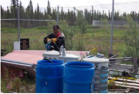
Pumping transformer liquids into 55-gallon drums. Beaver, Alaska
